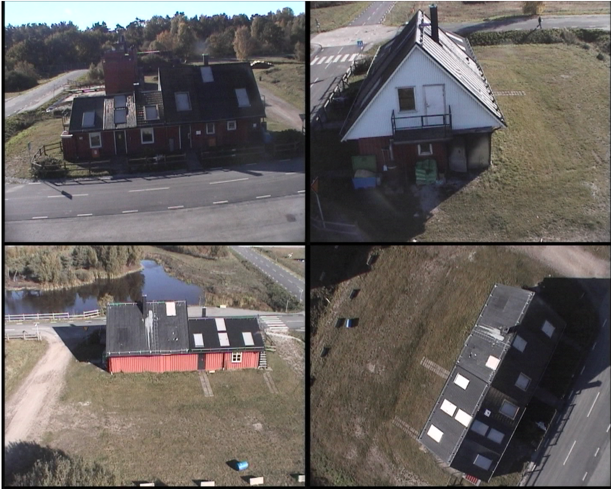
Figure 13: Mission 1. Images captured during the mission. Clockwise, starting from the upper left corner of the figure: the North, West, South and Top view of the building.
