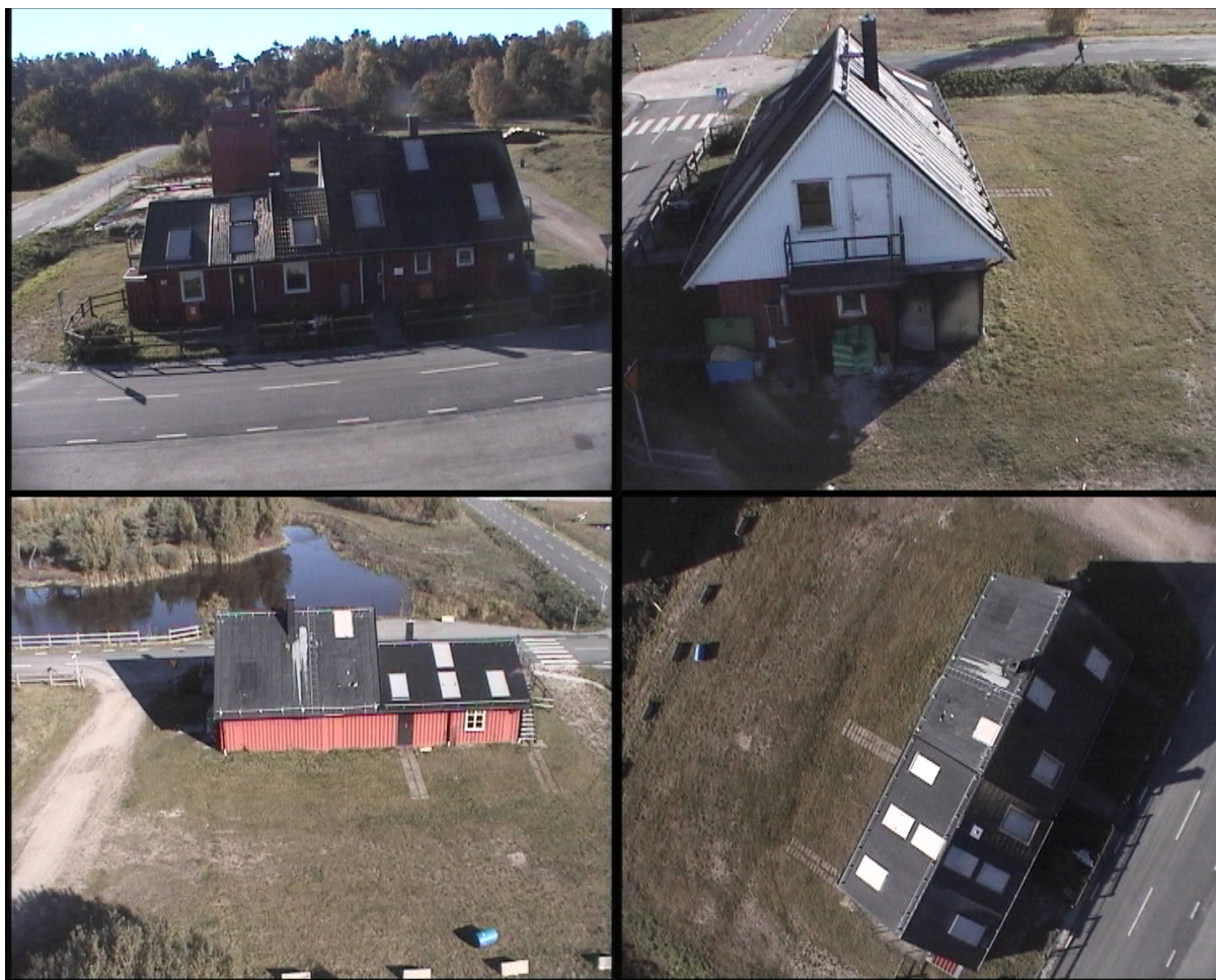
Figure 13: Mission 1. Images captured during the mission. Clockwise, starting from the upper left corner of the figure: the North, West, South and Top view of the building.
